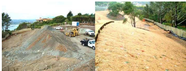
Before & after shots of erosion control upgrades
